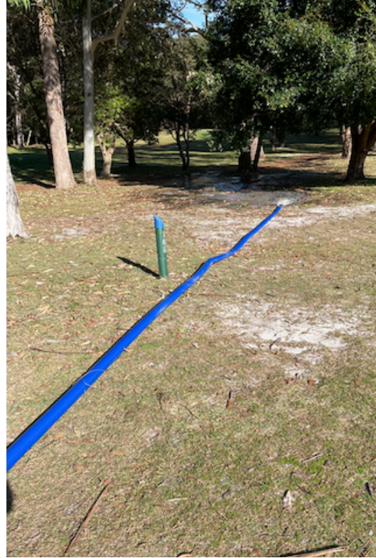
Mainline being flushed
