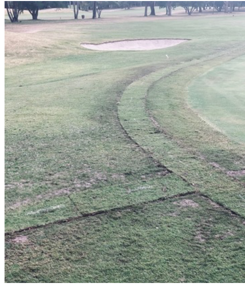
Completed work on the 3rd green
